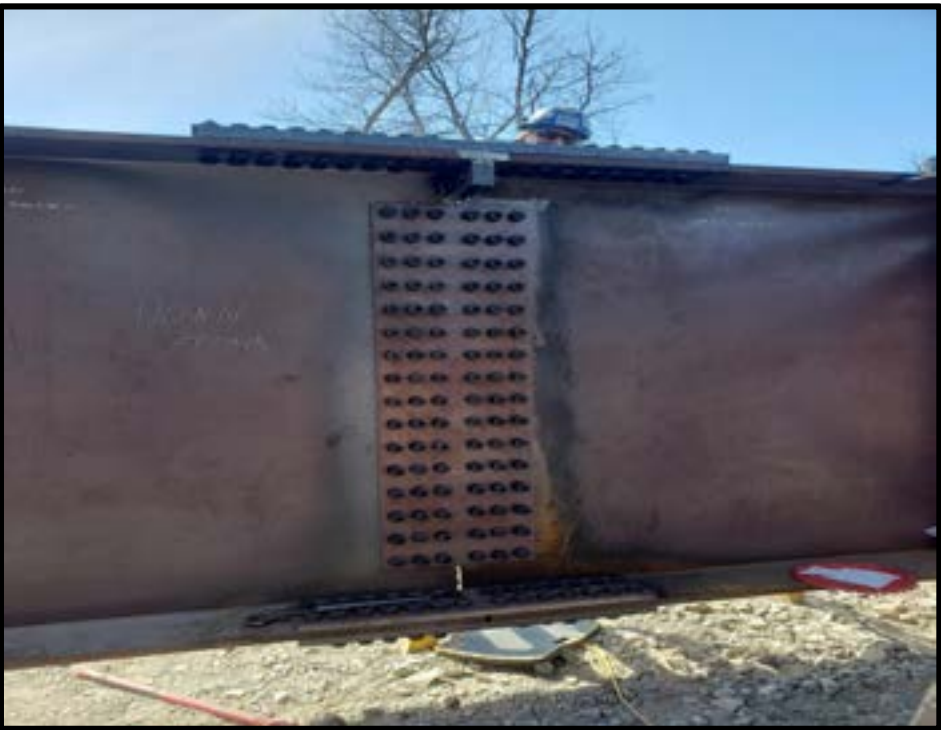
Photo 2 – splice bolts installed and snug tight, Apr 19.
