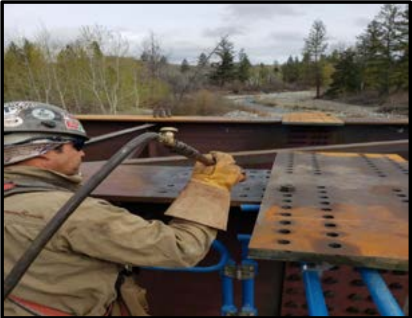
Photo 13 – Nelson stud installation prep, Apr 25.
