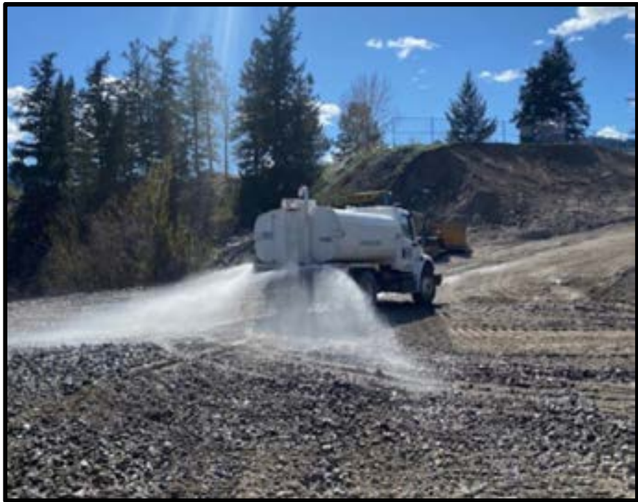
Photo 8 - watering west side where SGSB was placed, Apr 22.
