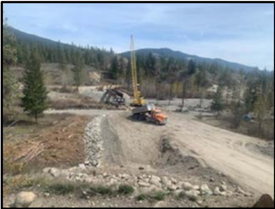
Photo 10 - hauling 75mm SGSB for placement on west abutment, Apr 23.
