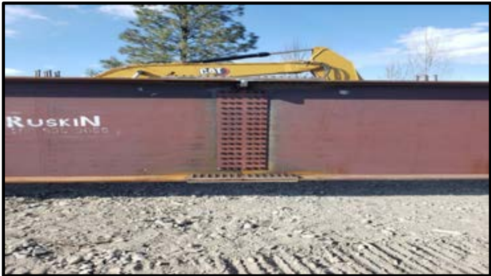
Photo 3 – web splice bolts installed, Apr 19.
