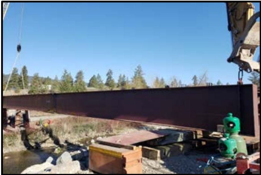
Photo 5 – Bridge span in location east abutment to pier, Apr 20.
