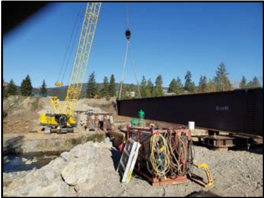
Photo 4 – Hoisting span into location on east abutment, Apr 20.
