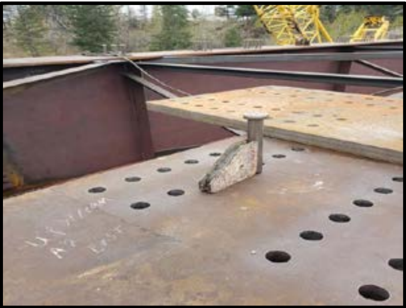
Photo 14 – First nelson stud installed, Apr 25.
