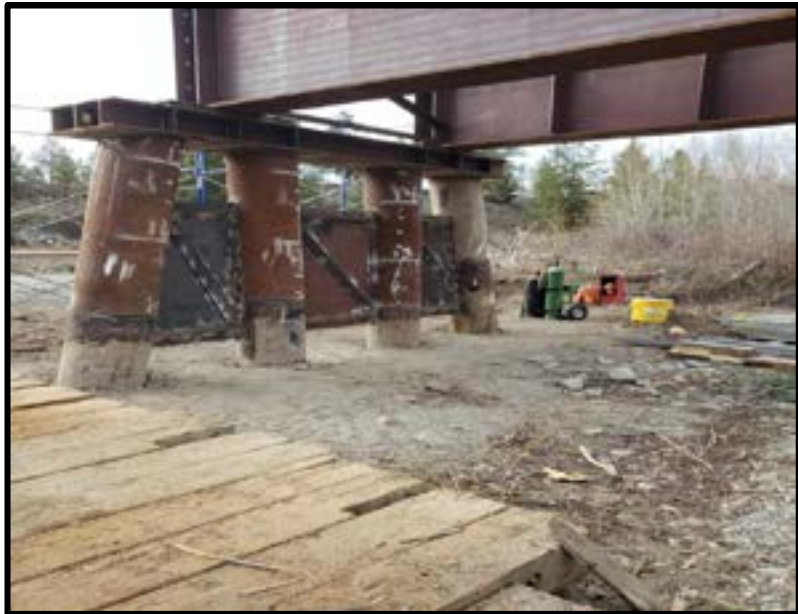
Photo 7- bearings to east cap welded and installed side-guides on bearings, Apr 20.
