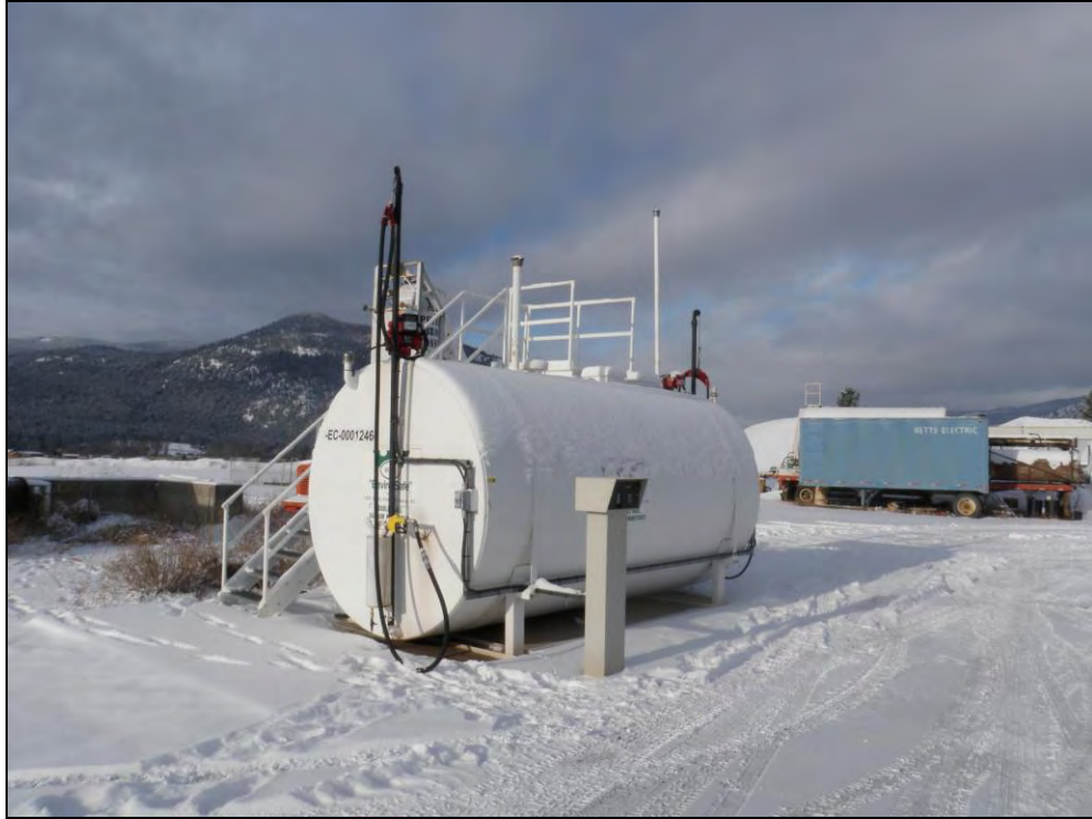
Photo 11. View of the 3000L Diesel AST (APEC 6) facing southwest.
