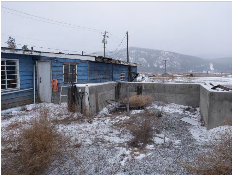
Photo 8. View of the dismantled former batch concrete plant at the back (west) side of the former Mojors service station (APEC 4), facing south.
