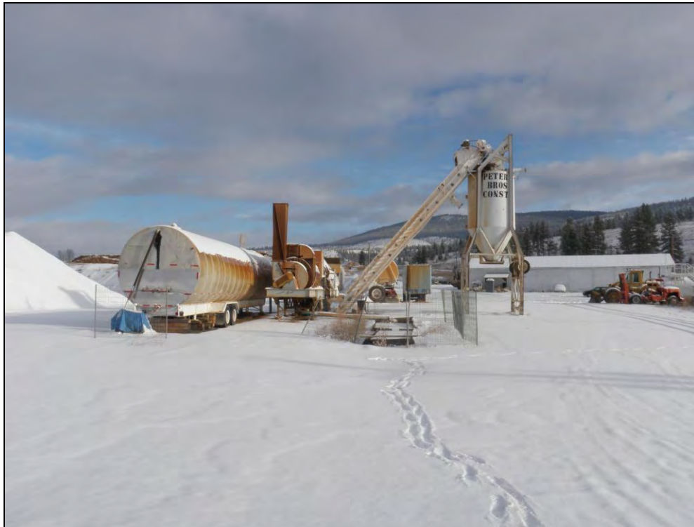
Photo 1. Overview of the Peter Bros Asphalt Plant (APEC 1) facing north.
