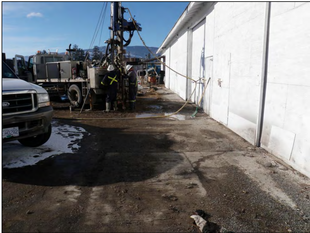
Photo 10. View of the broken concrete apron, minor soil staining on the south side of the warehouse (APEC 5) and BH2 facing west.
