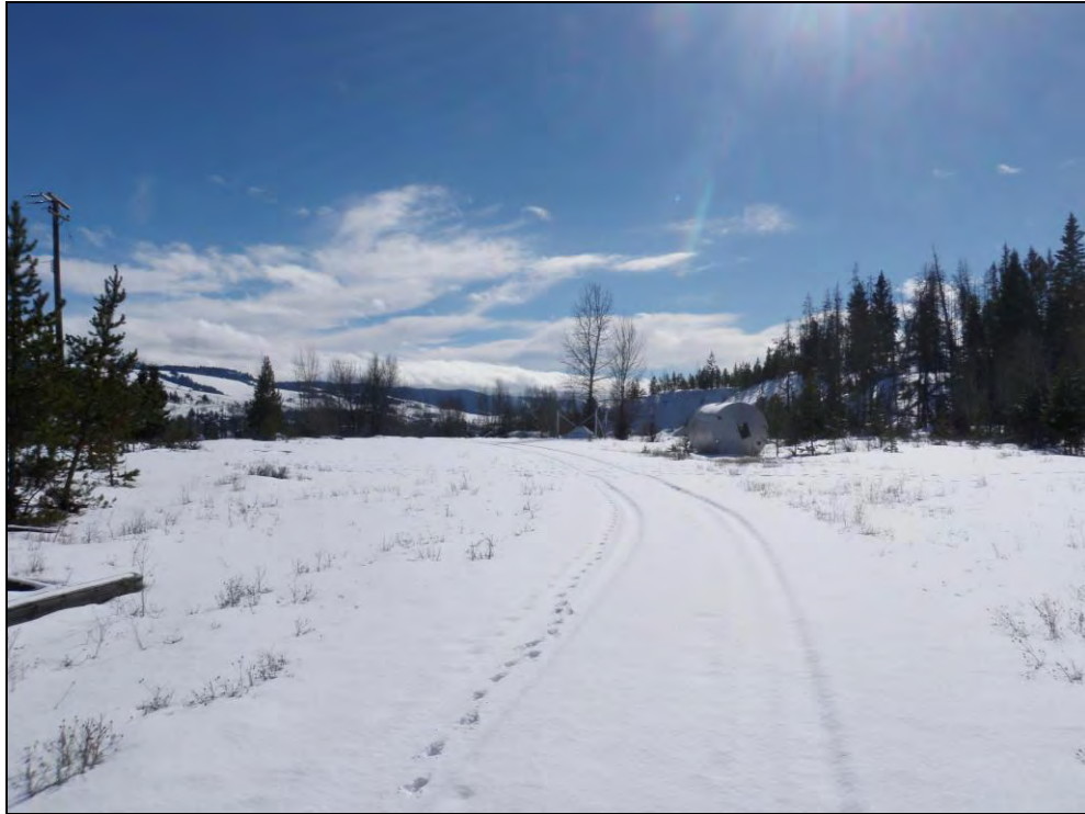
Photo 1. Overview of the Pipseul IR#3 Former Concrete Plant facing south. Note the collapsed silo (APEC 5).
