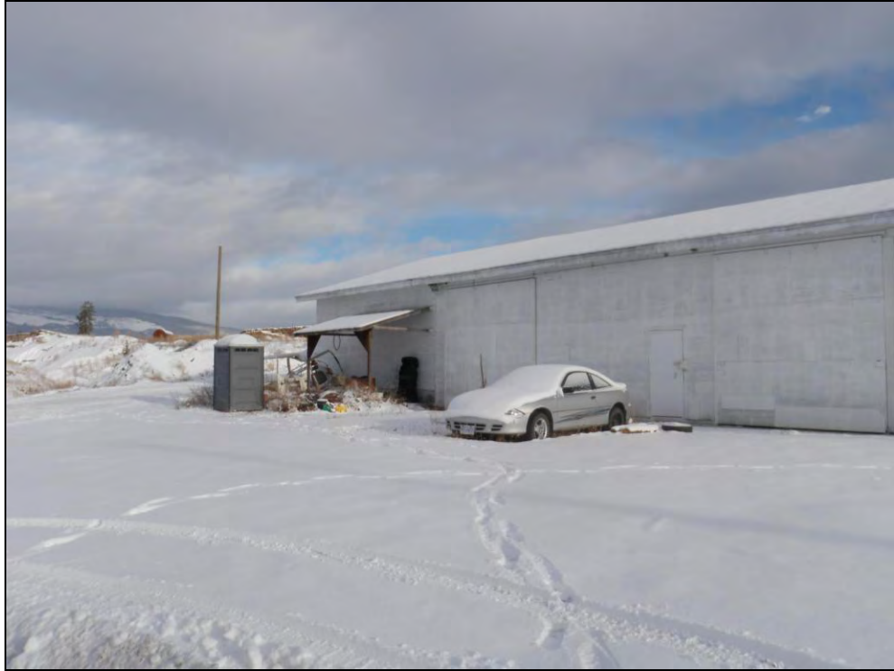
Photo 9. View of the former Mojo's Maintenance Building / Current Warehouse (APEC 5) facing north.
