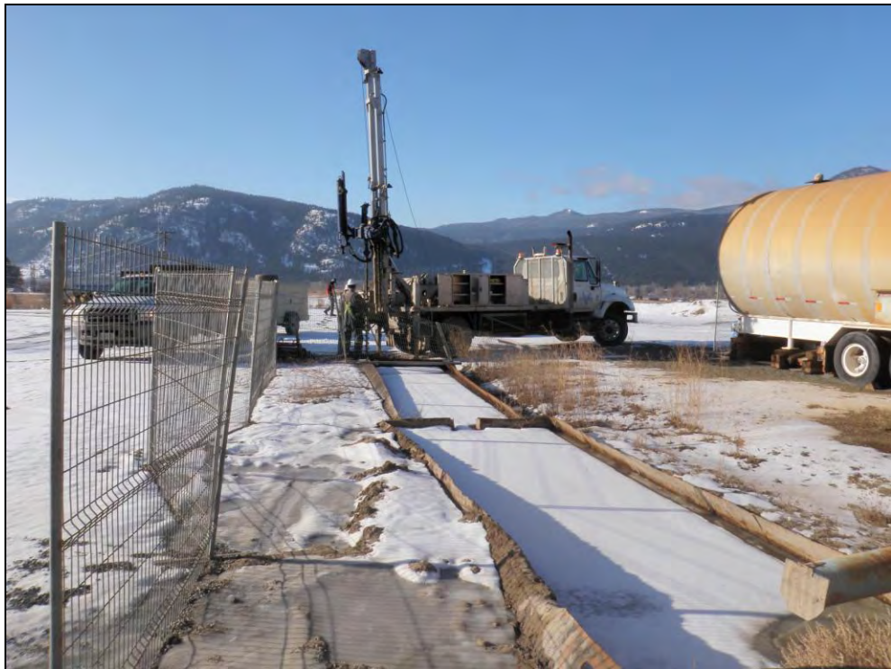
Photo 4. View the in-ground lined sumps at the asphalt plant (APEC 1) showing the location BH1 and MW14-1, facing south.
