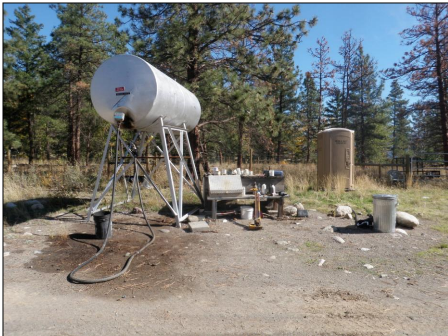
Photo 12. View of the Lot 2 AST (3221 Mill Creek Road) facing east. Note the soil staining below the tank, weeping valve, and adjacent hydrocarbon storage.
