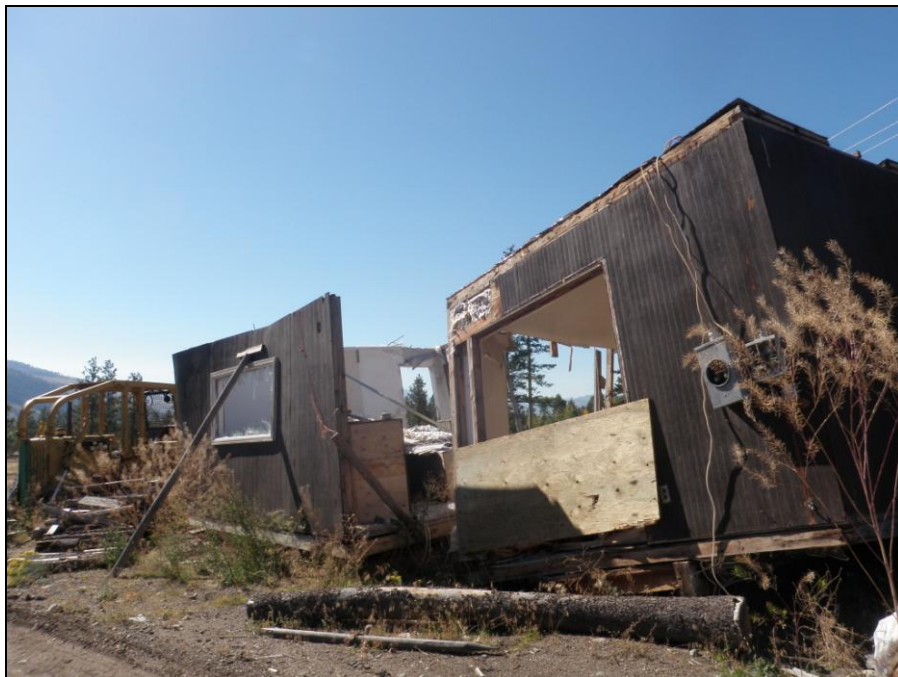
Photo 8. View of the collapsed office building and abandoned conveyor belts on the southwest portion of the Plan 59794 Post Mill facing south.
