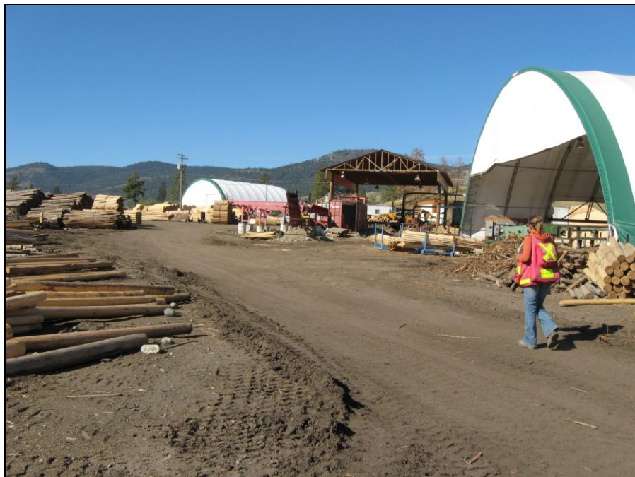
Photo 2. Overview of the post processing area (de-barkers, post point areas) on the northern portion of the Site (Plan 59794 Post Mill) facing west. Note the canvas covered buildings hold machinery for cutting, shaping, and trimming posts.
