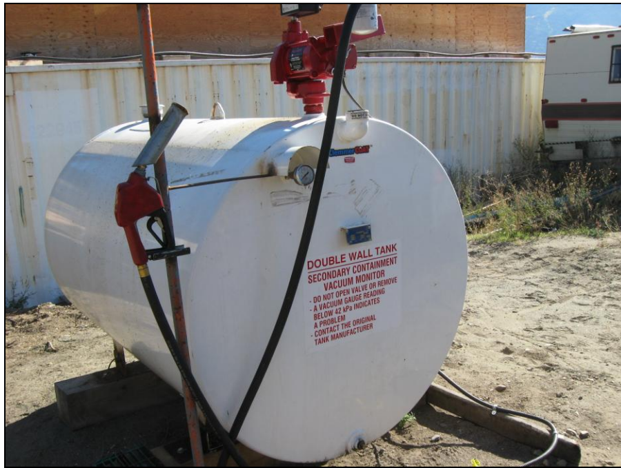
Photo 4. View of the new AST at the Plan 59794 Post Mill facing southeast. Note the travel trailer and oil storage area in the top right.
