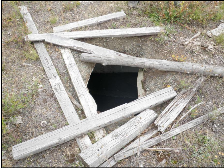
Photo 5. View of a sump located 30 meters west of the silo. The sump contained less than a meter of water with no detected odor or sheen.
