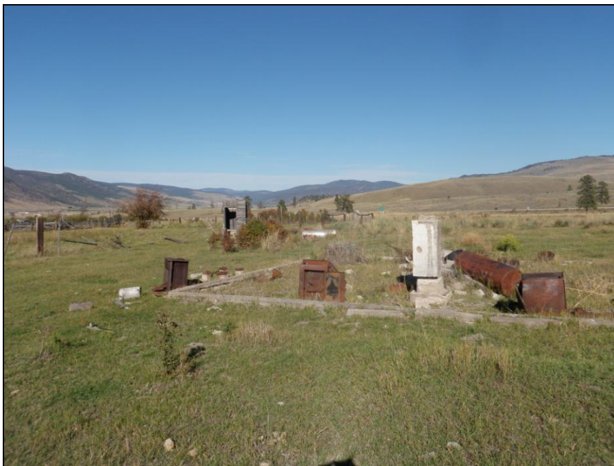
Photo 2. View of the Joeyaska IR2 Lot 9 Burnt House facing northeast. Note the occasional metal debris, concrete foundation, AST, and remaining chimney.
