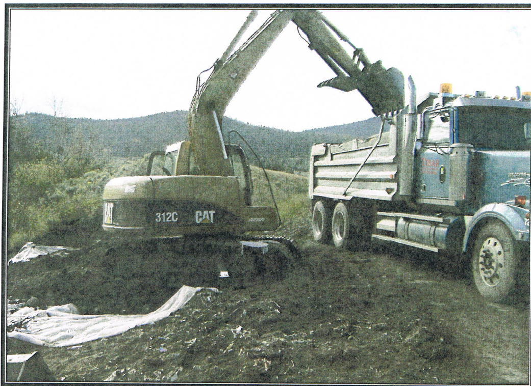
Photograph 6: Loading the trucks for offsite disposal of the contaminated material (9 Sept 2010).
