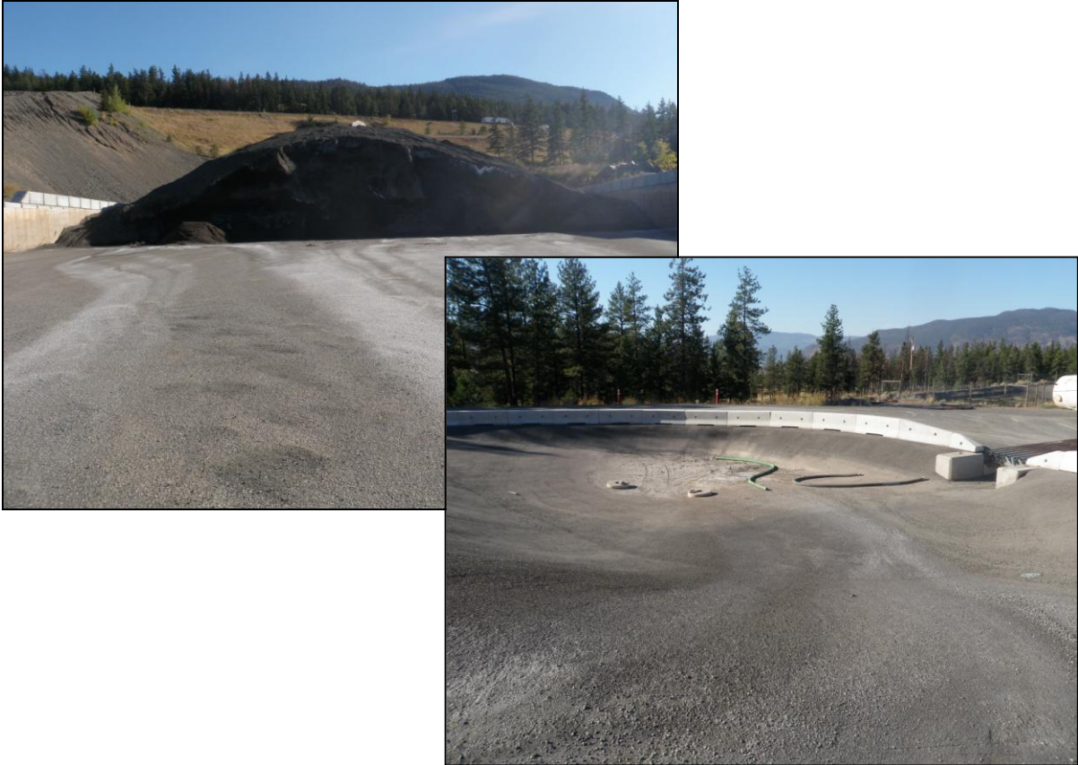
Photo 5. View of the used road salt pile (top left) looking south, and the concrete lined drain pit (top right) down gradient from the salt pile looking northwest at the Godey Gravel Pit. Note the salt staining on the concrete leading to the drain area.
