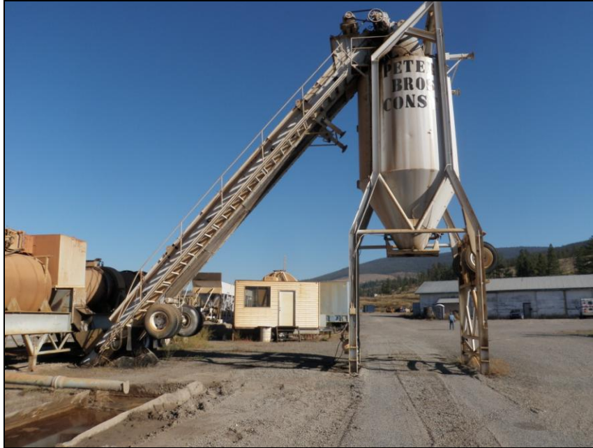
Photo 25. View of the asphalt silo, holding tanks, and office within the portable asphalt plant at Mojo's Gravel Pit facing north.
