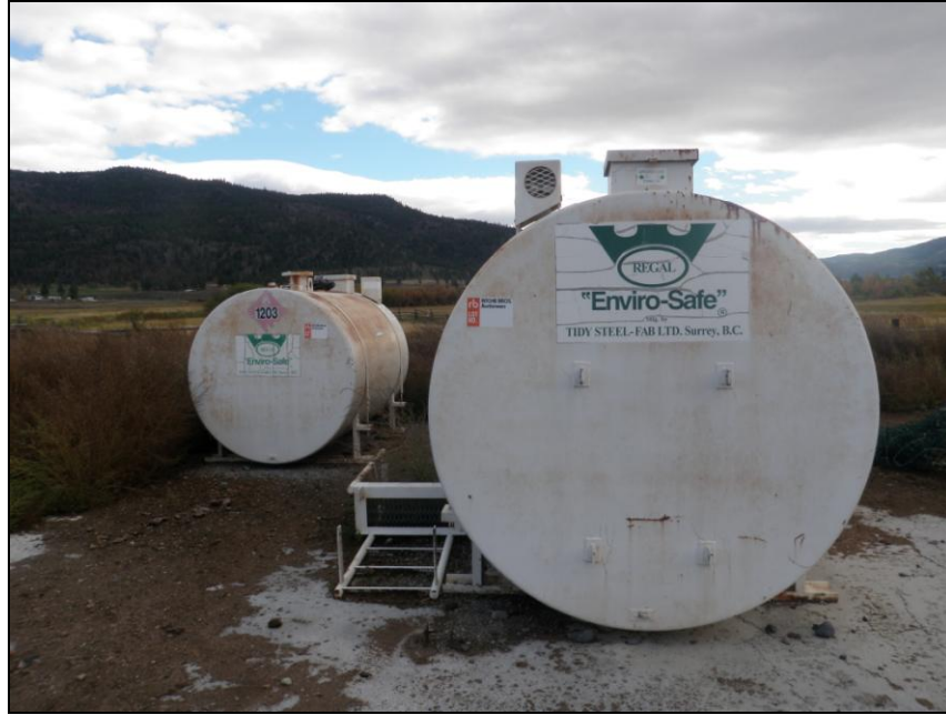
Photo 47. View of the Lot 183 Abandoned Gas Station ASTs facing east. Note the ASTs are empty and abandoned on a concrete pad south of the “Johnny’s on the Rez” Gas Station.
