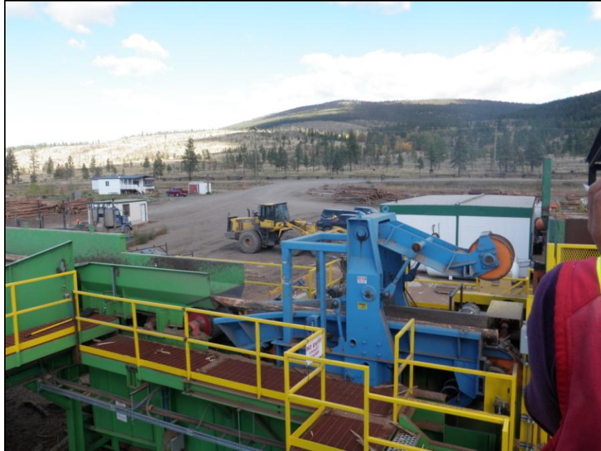
Photo 19. Overview of the sawmill de-barker (left) and conveyor to chipper facing northeast. Note the weigh scales and night watchman residence on the left, and the lunchroom on the right.
