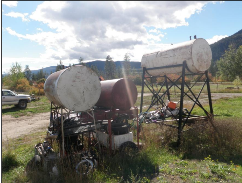
Photo 57. View of the Lot 200 ASTs on Fyall Road facing southeast. Note the lack of secondary containment and the moderate tank condition.
