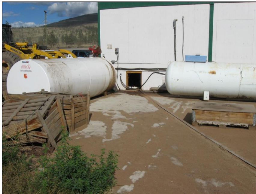
Photo 20. View of Lot 146 Sawmill ASTs (Diesel on left, propane on right) facing northeast. Note the concrete pad, and position next to lunchroom.
