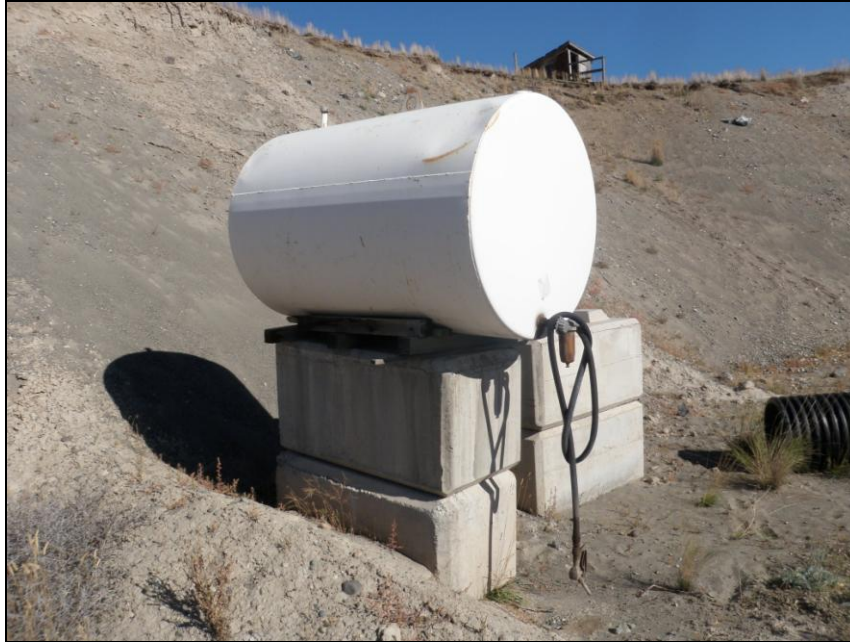
Photo 35. View of Lot 208 AST (213E) on Highway 8 facing northeast. Note that tank is likely to be moved to a more permanent location near the residence to the east.
