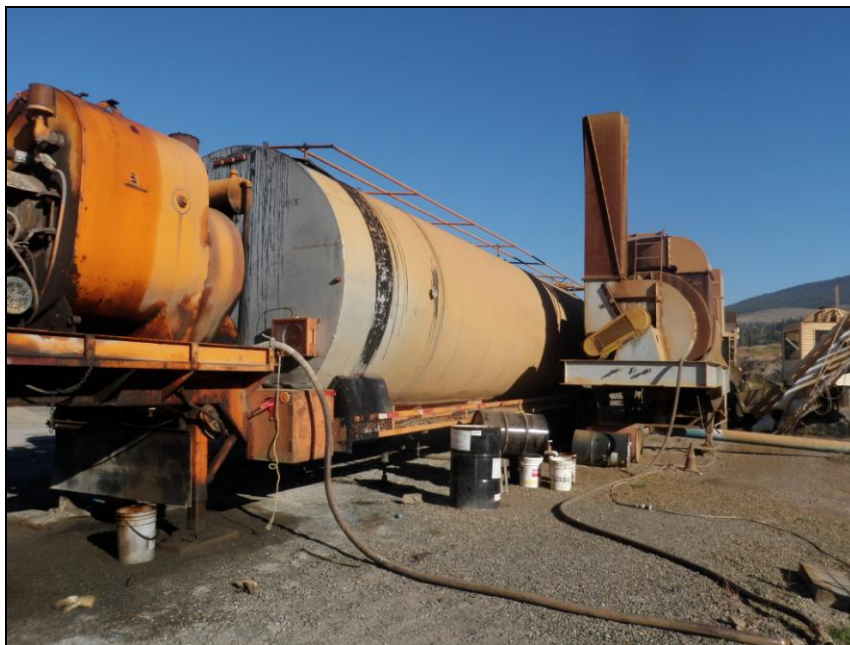
Photo 24. View of the portable asphalt plant at Mojo's Gravel Pit facing north. Note the 205L drums and 20L plastic pails and staining of soil beneath the machine. Stained area is lined with poly 30cm below the surface.
