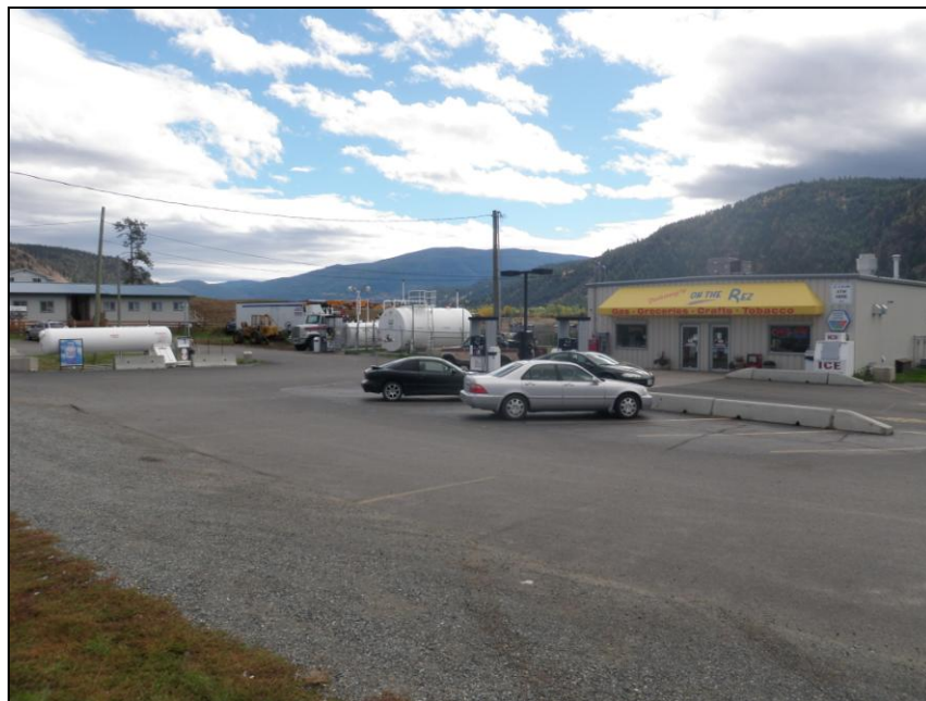
Photo 44. View of the Lot 78-2 “Johnnys on the Rez” gas station facing southeast. Note the pump island, store, propane, diesel and gas ASTs, and paved parking lot.
