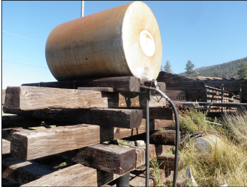
Photo 37. View of the Lot 58 AST (260E) on Highway 8 facing north. Note the treated wood supports, and second empty tank abandoned in the grass to the right.
