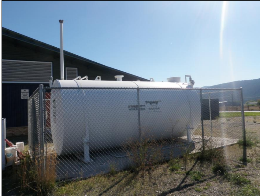
Photo 55. View of the LNIB School AST facing southeast. Note the concrete pad with the fenced compound.
