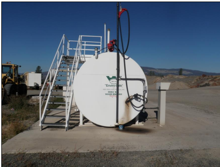
Photo 26. View of Lot 265 Mojos Gravel Pit Diesel AST facing west. Note the staining on the concrete pad.
