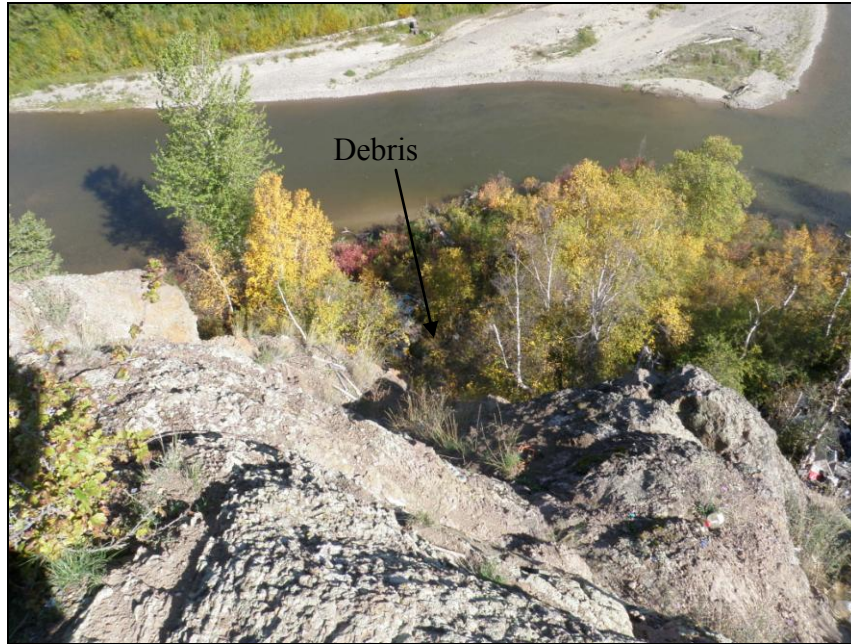
Photo 39. Overview of BC Plan 215 Nicola River Dump facing north. Note the debris scattered down the steep talus slope and close proximity to the Nicola River.
