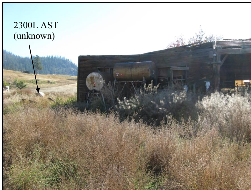
Photo 36. View of Lot 208 ASTs (225E) located on Highway 8, facing east. Note the Diesel and Gas AST against the collapsing building, and the unknown AST on a wood pallet in the field.
