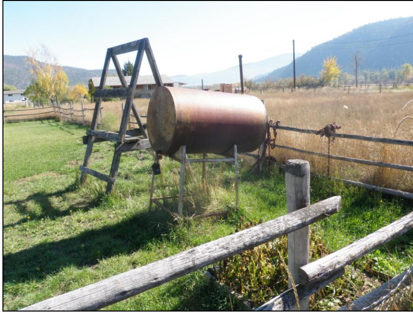
Photo 51. View of the Lot 12 AST facing east. The rusted tank and appears empty and without secondary containment.
