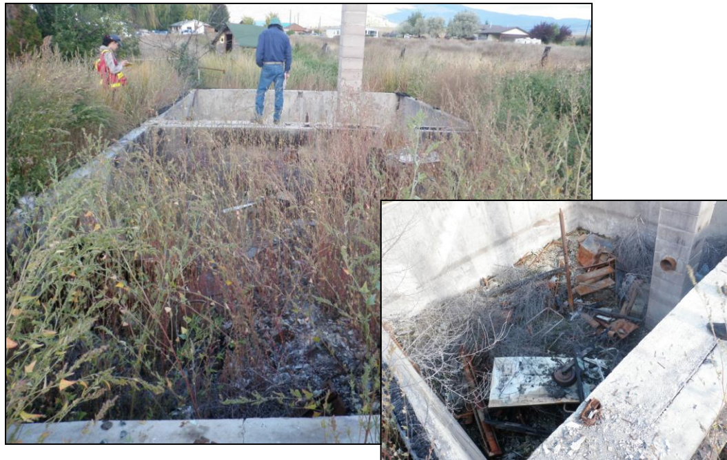
Photo 48. View of the Lot 81 Burnt House concrete foundation facing west. Note the burnt debris and standing water within the basement (shown on right), and the wooden shed to the west.
