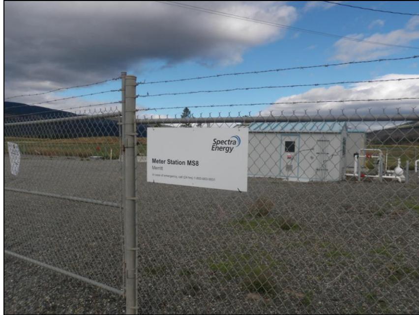
Photo 43. View of the Lot 96 Spectra Energy Power Station located off reserve facing northwest. Note the three meter station buildings, and pesticide use notice on the fence at left.
