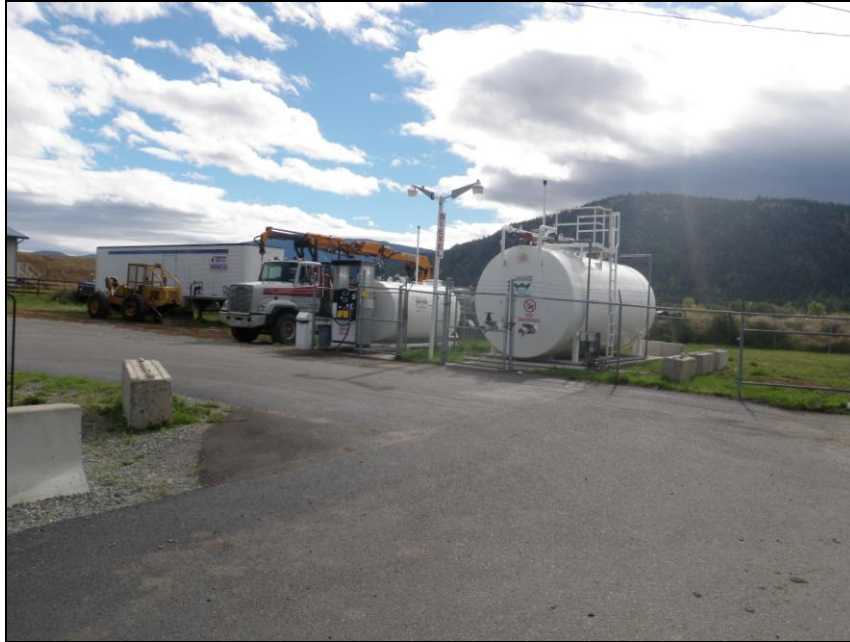
Photo 45. View Lot 78-2 “Johnnys on the Rez” gas station ASTs facing south. Note the two ASTs (Diesel at left, Gas at right) are on concrete pad within fenced compound. Note minor diesel staining on concrete below nozzle.
