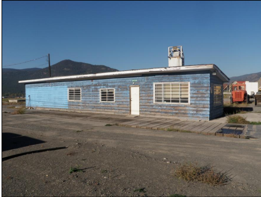
Photo 23. Overview of the abandoned Mojos Gas Station Building on Lot 265 facing southwest. Note the sump below the treated wood at the front of the building, and remaining concrete pad.
