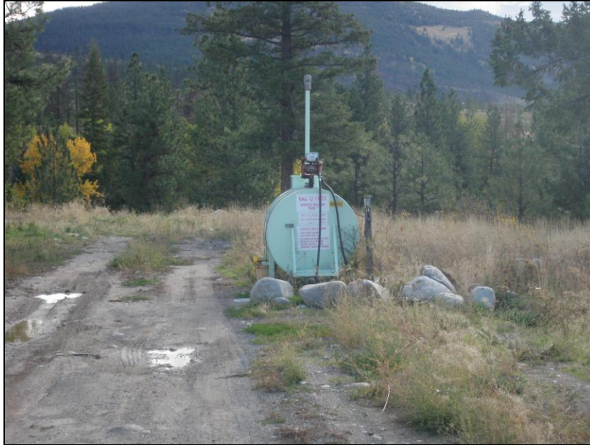
Photo 5. View of the Lot 254 AST facing east. Note the lack of secondary containment, and good tank condition.
