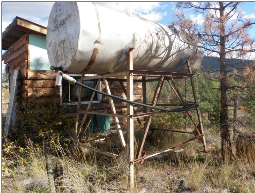
Photo 6. View of the empty Lot 279 AST facing northeast. AST is not in original fueling location with a slight rusting and peeling on tank.
