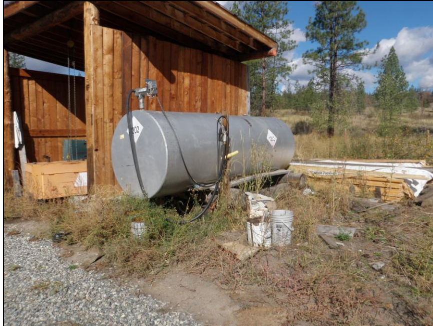
Photo 3. View of the Lot 219 AST facing northwest.
