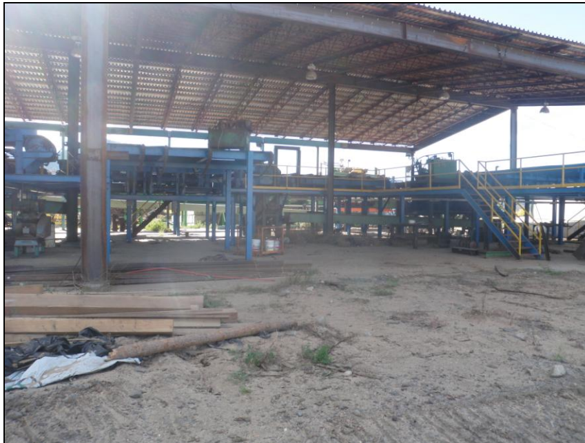
Photo 22. View of the inoperable sawmill, and limited petroleum product storage within the covered building. Note the concrete pad below.
