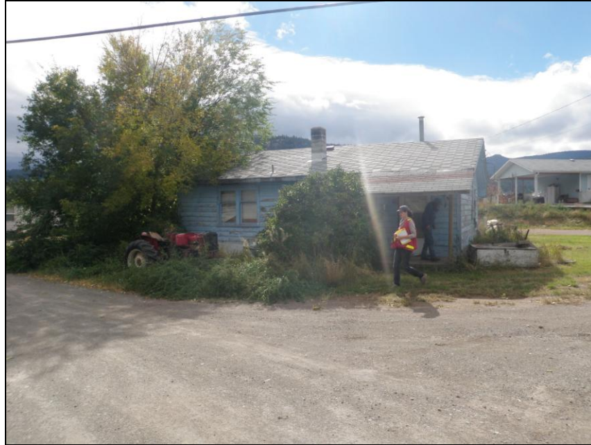
Photo 33. View the Lot 72-1 Abandoned House facing south. House reportedly contains xenolite (asbestos) insulation.
