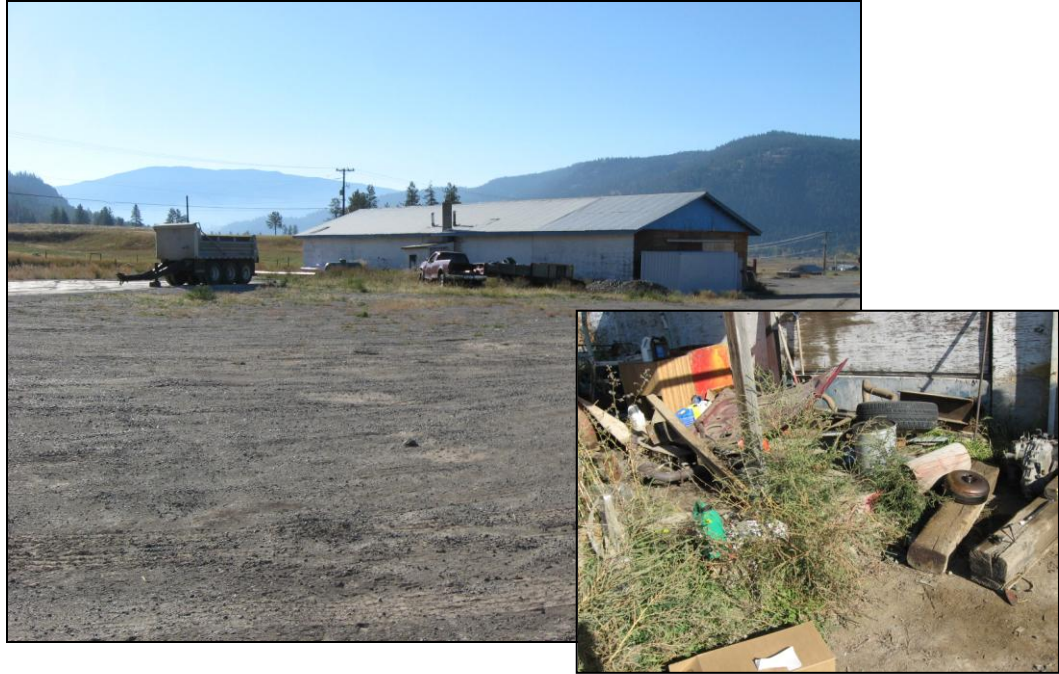
Photo 27. View of the warehouse within the gravel pit facing south. Debris and the storage of automotive lubricants and oil are found outside the warehouse.
