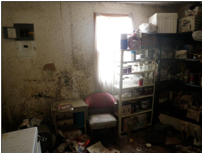
Photo 30. View of the interior of the Lot 105 Abandoned House showing mold on walls, and remaining household materials inside.
