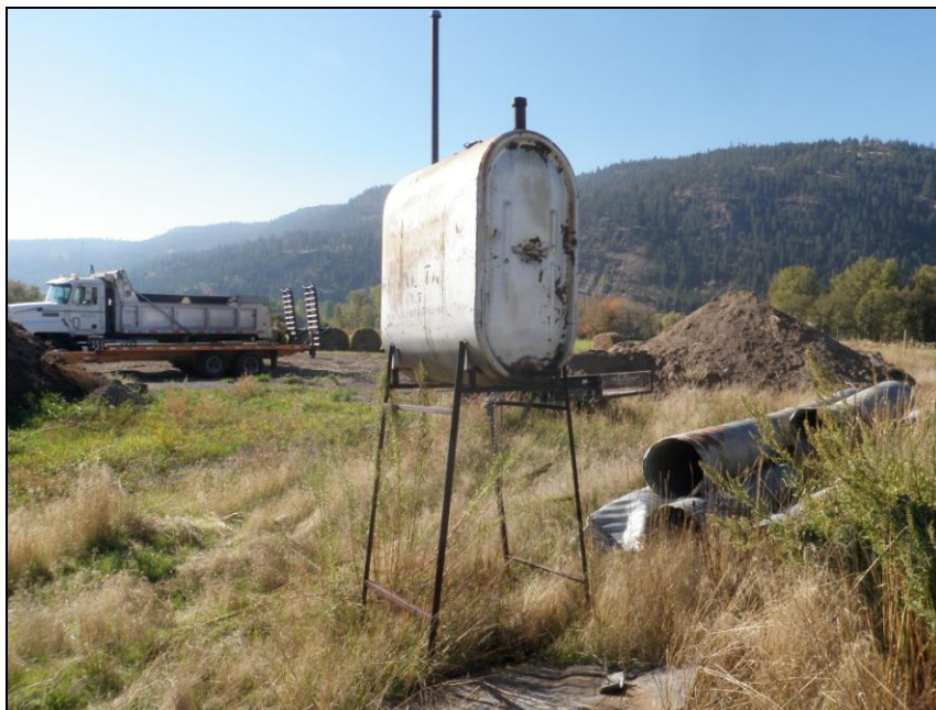
Photo 38. View of Lot 58 AST (280E) on Highway 8 at facing southeast. Note the lack of secondary containment, and no staining or odors.
