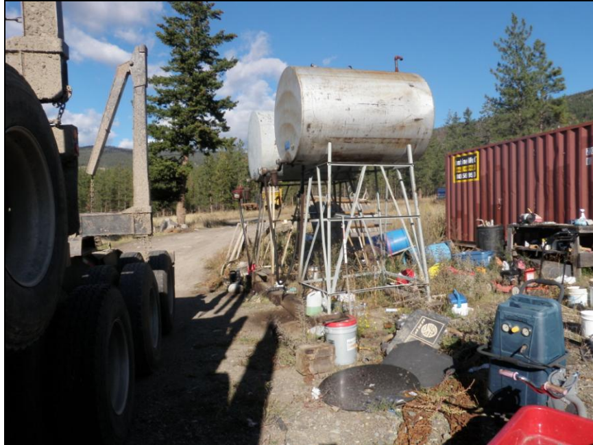
Photo 17. View of the two diesel ASTs located on Lot 294 facing northeast. Tanks appear in good working condition with some weeping at the bungs and fill pipes. Note the adjacent hydrocarbon product storage, and staining below tanks.
