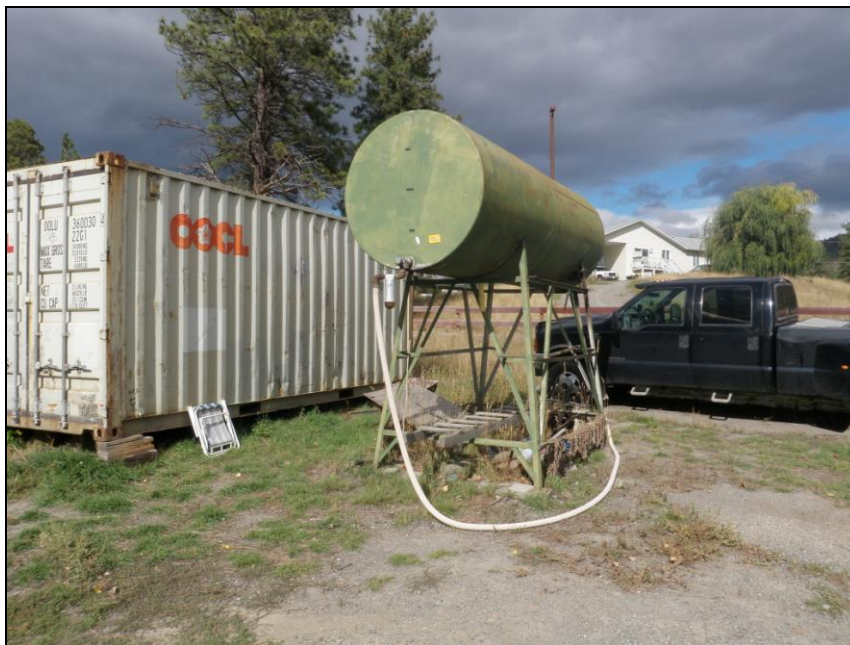
Photo 32. View Lot 87-4 AST facing north. Note small stain in soil below tank, and open 20L pail containing radiator fluid below tank supports.
